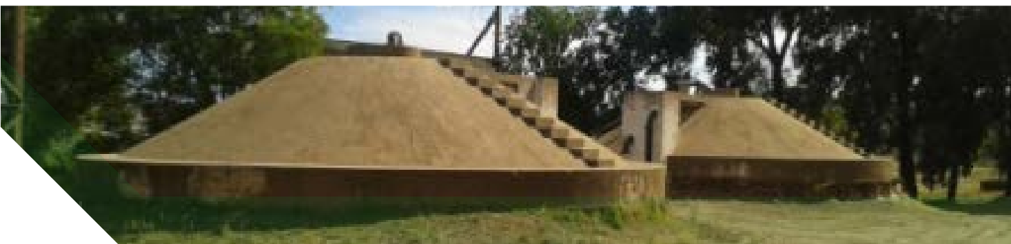
Digesters at Maletswai WWTW
