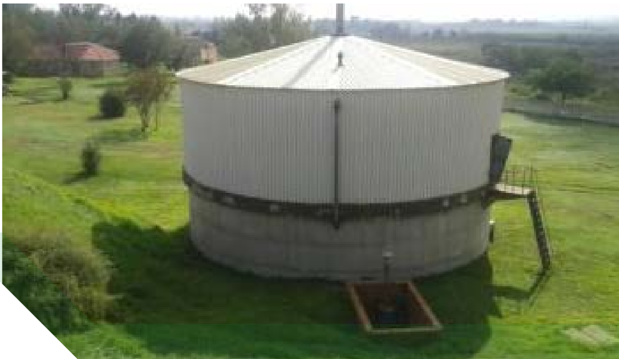
Existing 1000m 3 biogas storage tank
