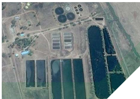
Google view of the Newcastle WWTW
