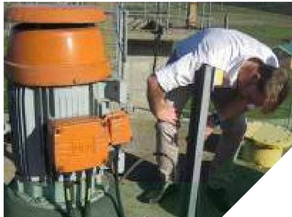
Inspection of the existing digester at the Gwaing WWTW
