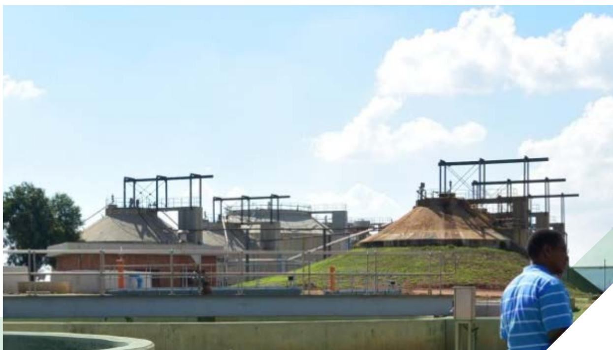
Digesters at Sunderland Ridge WWTW
