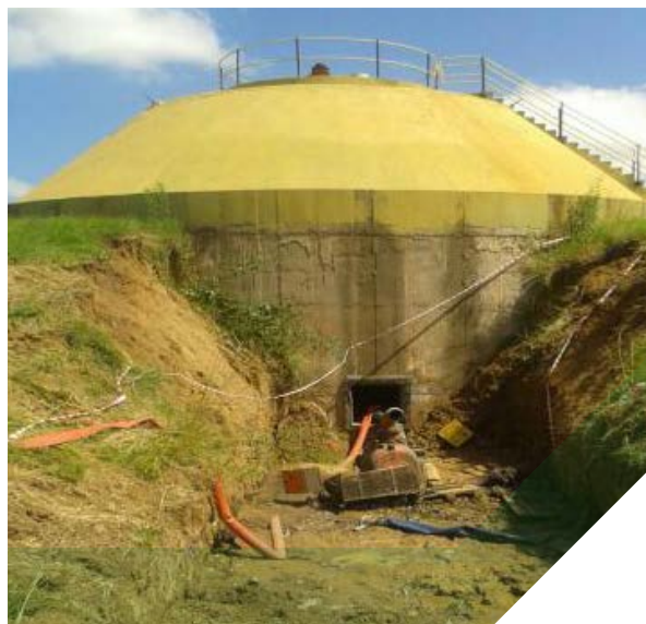
Digester being de-sludged
