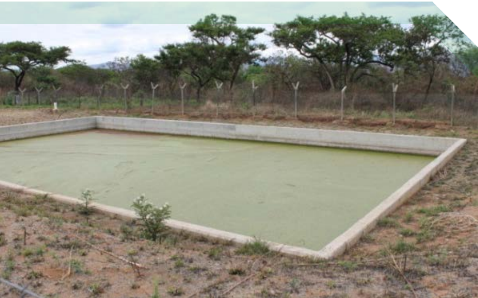
Sludge dam at Umjindi WWTW
