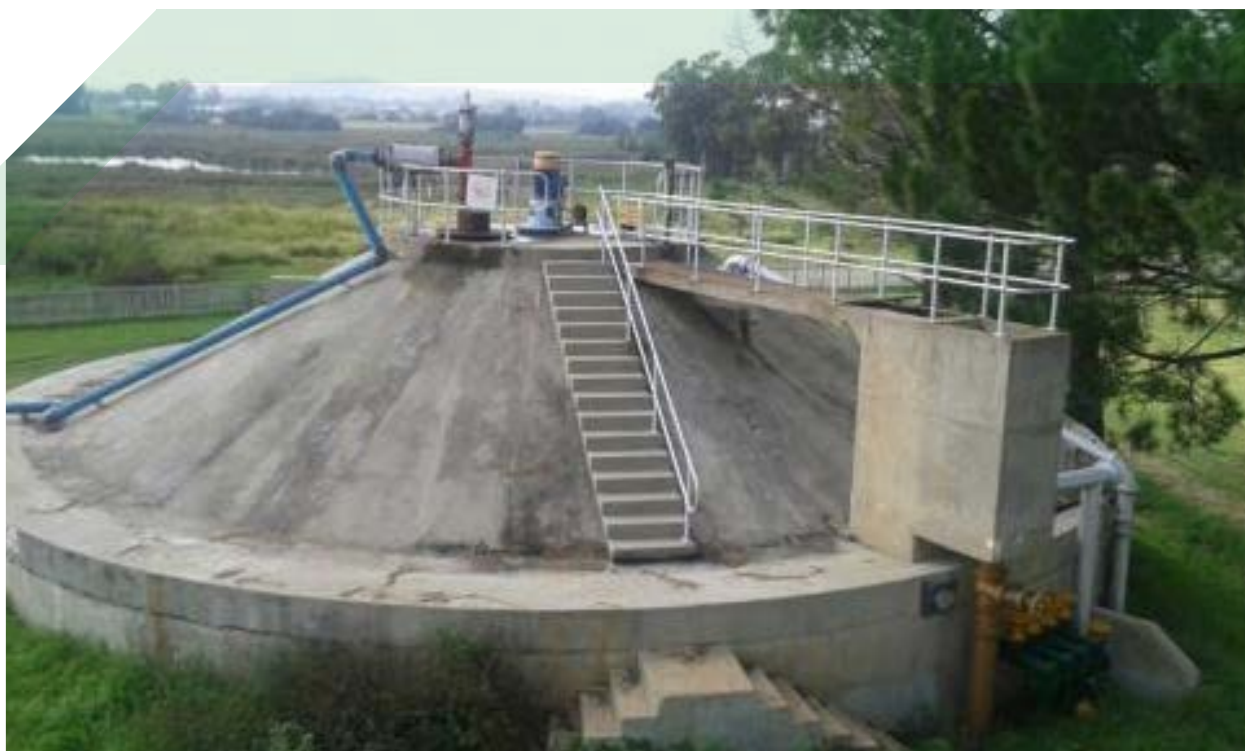
Existing digester at Tlokwe WWTW
