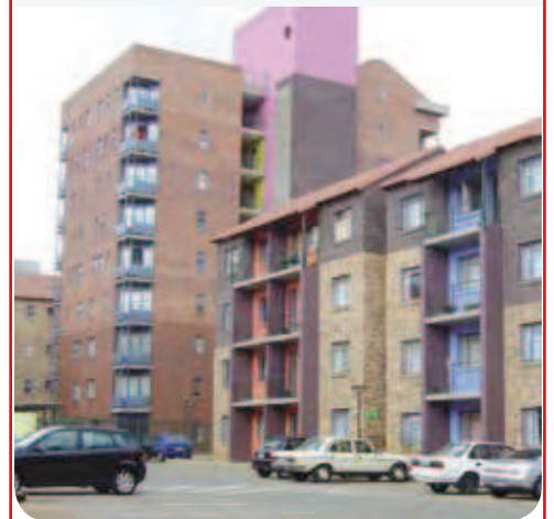
Variation in social housing blocks, Brickfields, Johannesburg
