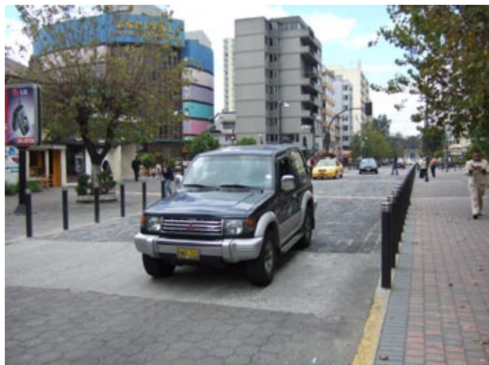
Fig. 13.29 Raised intersection in Quito.
