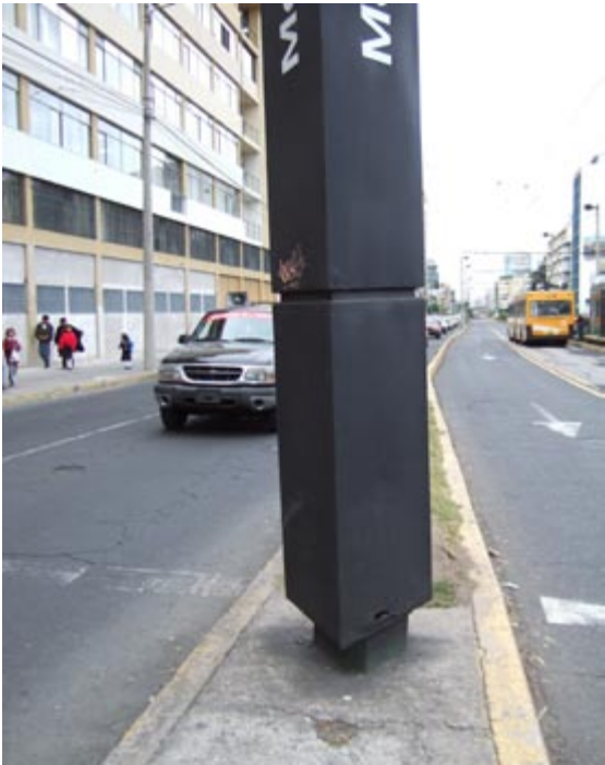
Fig. 13.61 This BRT identification post in Quito is placed in a pedestrian island, and acts to block the pedestrian’s view of both oncoming mixed traffic as well as oncoming BRT vehicles.
