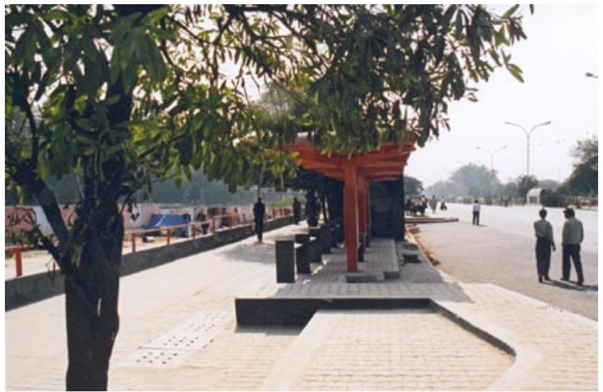
Fig. 11.78 ▲ Complete bus shelter with integrated vendor space.
