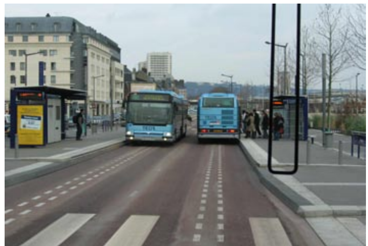
Fig. 12.43 and 12.44 The dotted white line along the lanes of the Rouen system permit an optical guidance system to manoeuvre the vehicles to a high degree of accuracy.
