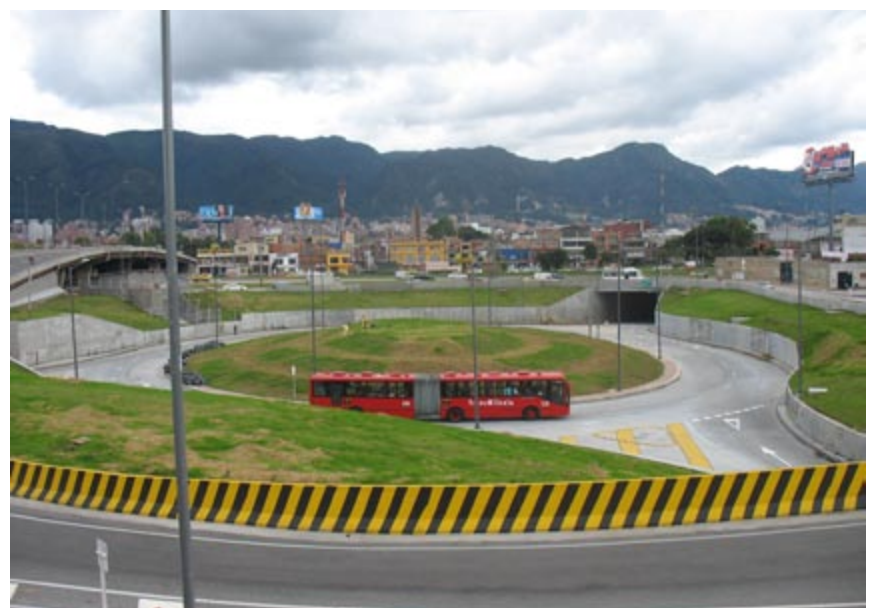
Fig. 9.34 At the major intersection of TransMilenio's Calle 80 (80 th Street) corridor and NQS corridor, a set of underpasses, a roundabout, and an overpass helps facilitate exclusive turning movements for BRT vehicles.
