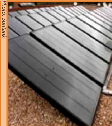
Solar water heating on retirement centre
