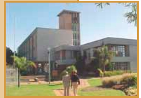
Tygerberg Administration building
