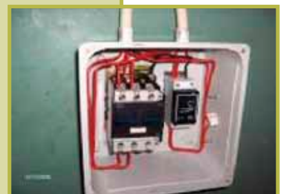
Lights timer set to switch on at 05h30 and switch off at 19h00
