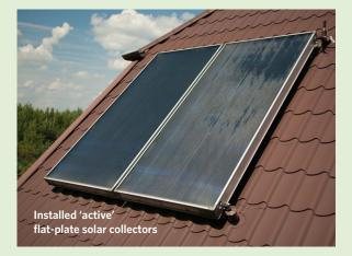
Flat plate or evacuated tube? A flat-plate system collects the sun's heat through a weatherproof box with a glass cover, whereas an evacuated-tube system does so through a series of parallel glass tubes. Evacuated-tube systems are designed for colder climates and typically reach higher water temperatures than flat-plate systems.
