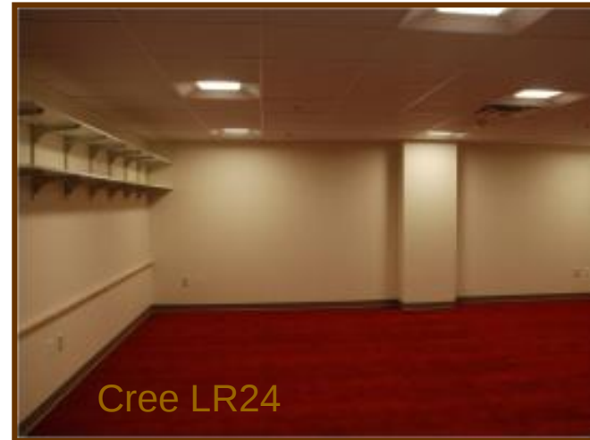
After: The same room at the Pentagon after Cree's LED lights were installed (Credit: Cree)
