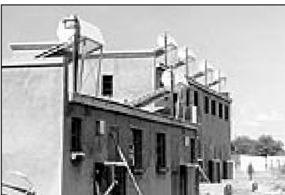
Above: Lwandle Hostels-to-Homes Project showing the solar water heaters.
