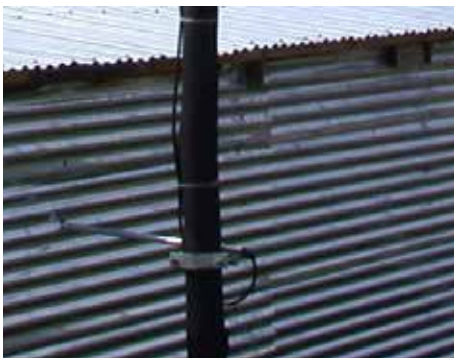
Municipal electricity connection for informal households showing service pole and prop from the pole to support the readyboard in the house
