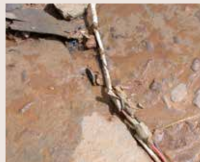
Illegal live electricity connection running across main access road and surrounded by water
