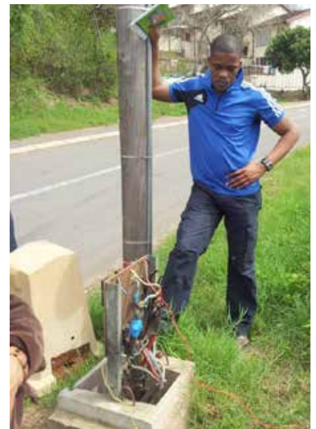
Example of an illegal electricity connection
