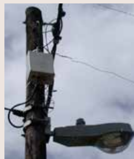
Taking illegal connection straight off the ABC
