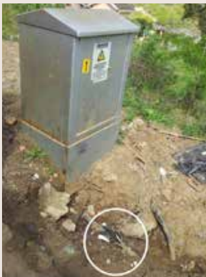
Illegal connections in a trench
