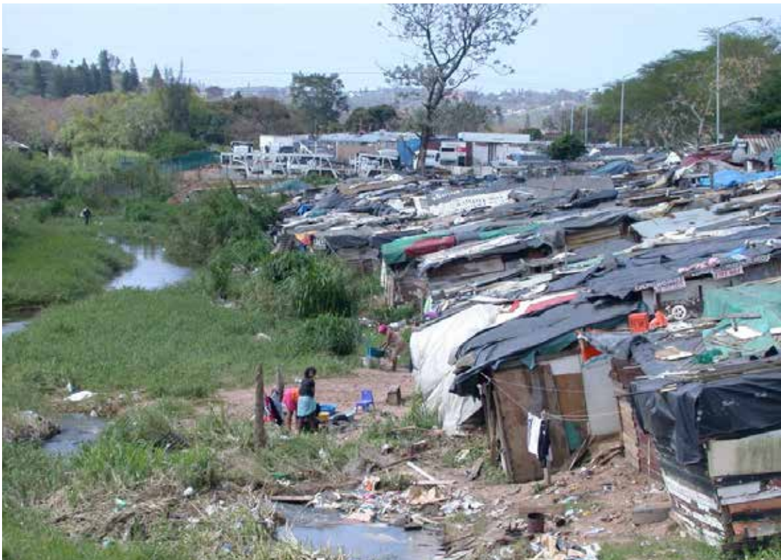
Part of this settlement is in a regularly flooded area in eThekweni municipality – can they can still be connected (they are already, but illegally and unsafely)?
