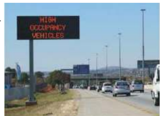
The Variable Message Service used to provide users of the N1 with information about the use of the HOV lane
