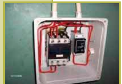
Lights timer set to switch on at 05h30 and switch off at 19h00
