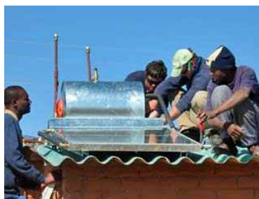
A solar water heater being mounted in Cosmo City
