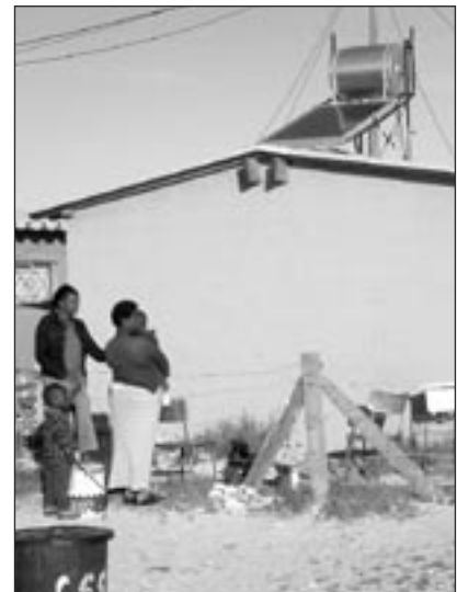
Above: At Kuyasa, solar water heaters were installed at 10 houses.
